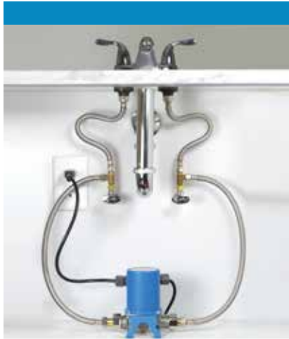
AMH1K-1 Kit Installed
